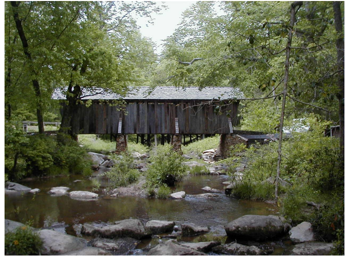
Pisgah Covered Bridge Asheboro, North Carolina
